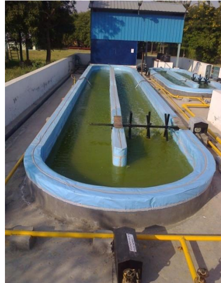
Microalgae Pilot Plant
